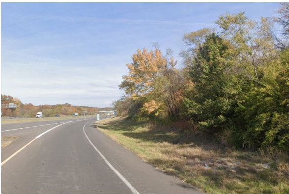
I-435 on-ramp at NE Shoal Creek Parkway
