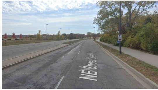
South on NE Shoal Creek Parkway
